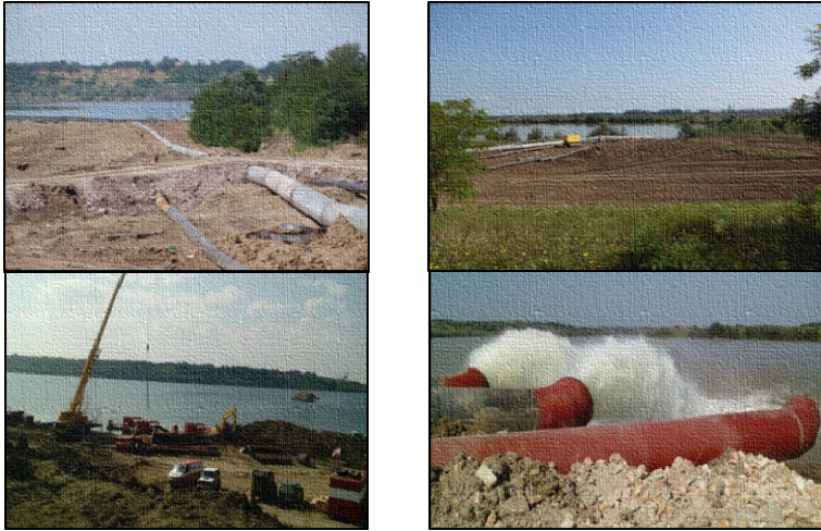
Figure 7 Prepare and begin pumping water from the pit Tamnava West field, RB Kolubara, (September 2014), R. Serbia, [4]
