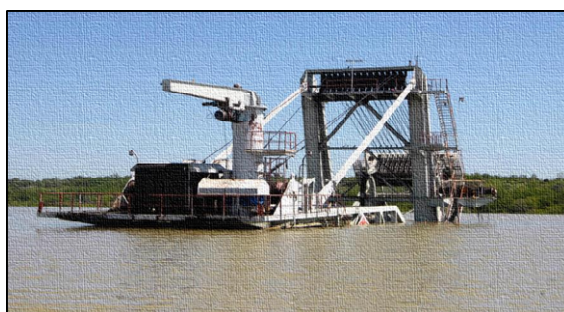
Figure 2 View of the flooded open pit mine Tamnava West field, RB Kolubara, (September 2014), The Republic of Serbia, [3]
